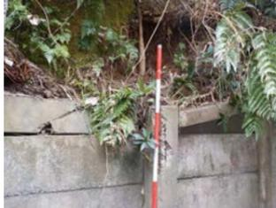
広幅かつ横断的な鉄筋が露出<br>
