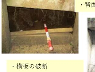
背面度露出、背後に空洞<br>
